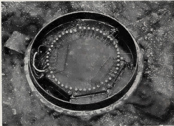
Fig. 175. Kabelfordelingshus (aaabent)
