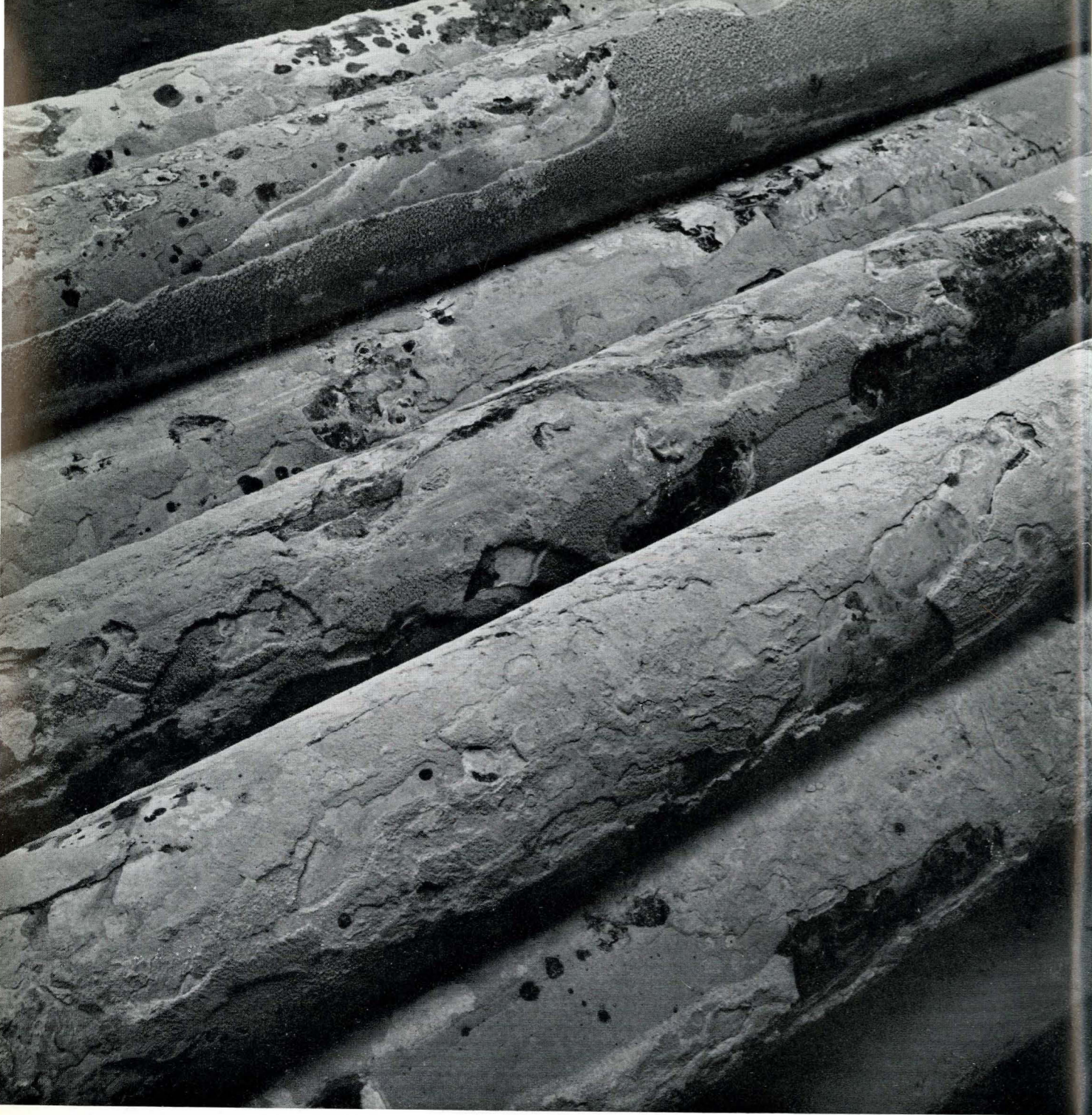
Temporary and permanent hardness are two causes of scale formation. They may also be responsible for corrosion. The photograph shows tubes from a Locomotive running on untreated water of medium hardness. Note thickness of scale and commencement of 'pitting'. London & North Eastern Railway Co., Ltd.
