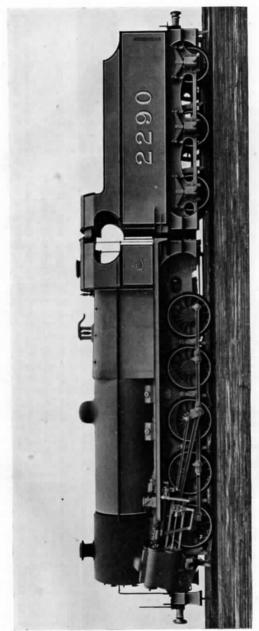
Fig. 263.—Four-Cyllinder 0-10-0 Banking Engine, L.M.S.R. The late Sir Henry Fowler, K.B.E., Chief Mechanical Engineer.
