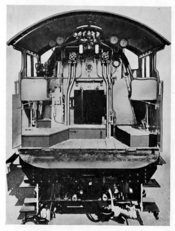
Fig. 62.—A Modern Locomotive Cab and Fittings (L.N.E.R. 4-6-2 Locomotive).
