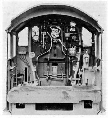
Fig. 272.—View of Footplate and Fittings: G.W.R. "KING" CLASS LOCOMOTIVE.
