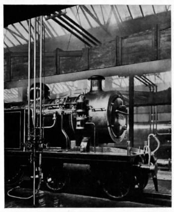
Fig. 4.—Washing Out a Locomotive Boiler by the Economical Hot-Water System.
