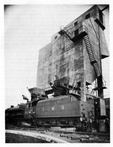
Fig. 14.—Mechanical Locomotive Coaling Plant at Preston, L.M.S.R.
