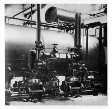
Fig. 3.—Example of Economical Single-Tank Hot-Water Boiler Washing-Out Plant.
