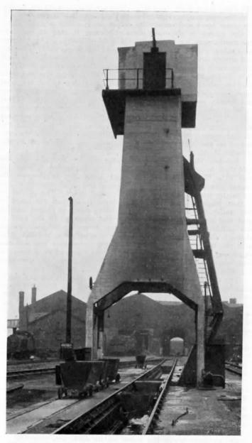
Fig. 17.—Coaling and Ash Plant at Kentish Town, L.M.S.R.
